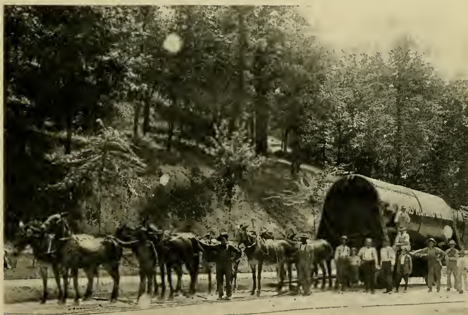
Moving a 60,000 pound Boiler over Hot Springs Mountain by Hot Springs Plumbing and Machine Company Contractors in all kind of Machinery Plumbing and Heating
